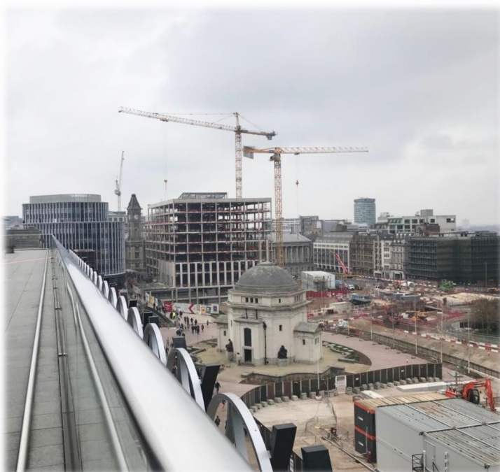
New infrastructure development, Birmingham
