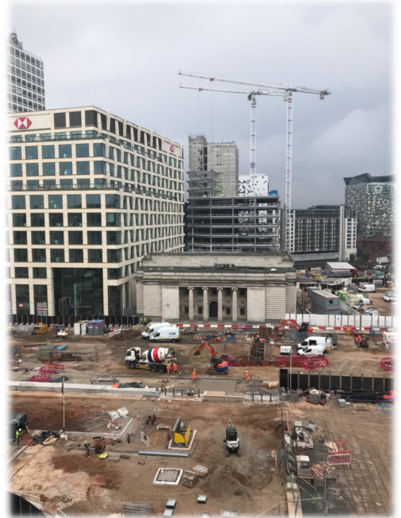
New infrastructure development, Birmingham
