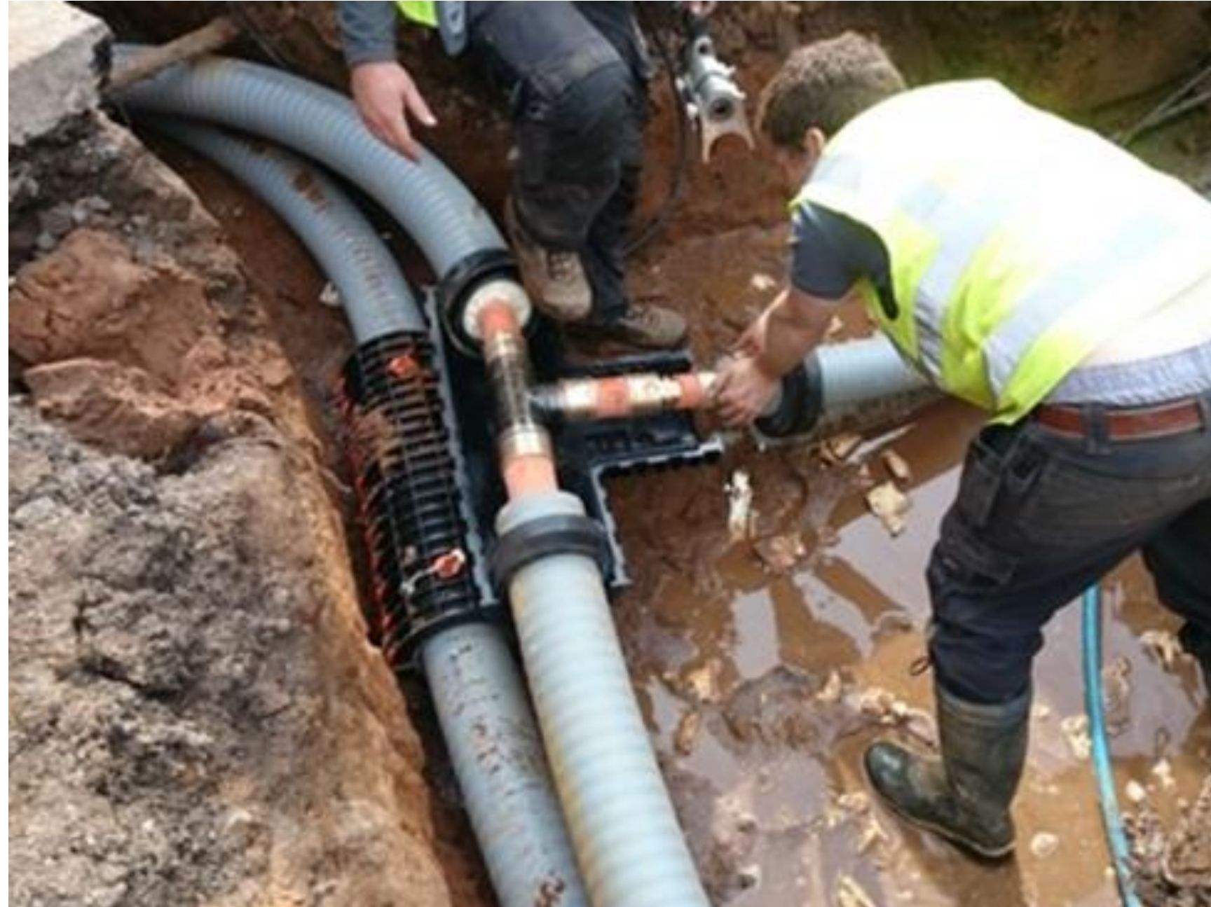
District Heat Main Installation, Cumbria
